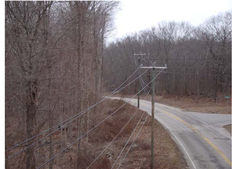
After enhanced tree trimming
