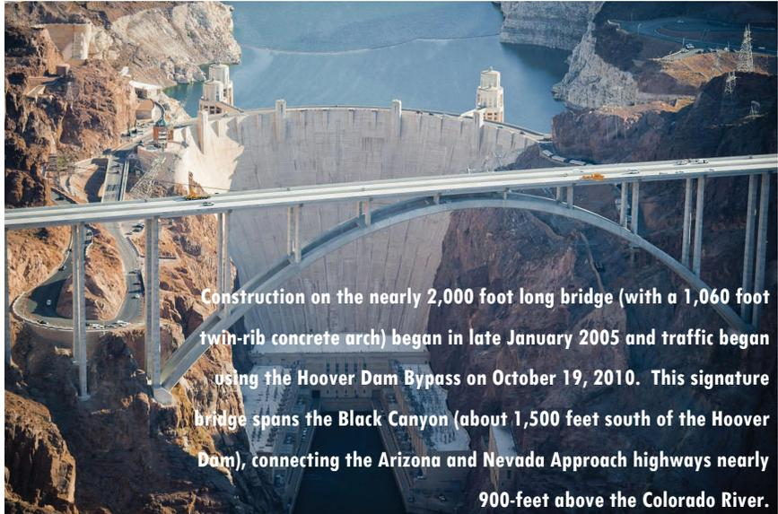
Construction on the nearly 2,000 foot long bridge (with a 1,060 foot twin-rib concrete arch) began in late January 2005 and traffic began using the Hoover Dam Bypass on October 19, 2010. This signature bridge spans the Black Canyon (about 1,500 feet south of the Hoover Dam), connecting the Arizona and Nevada Approach highways nearly 900-feet above the Colorado River.
